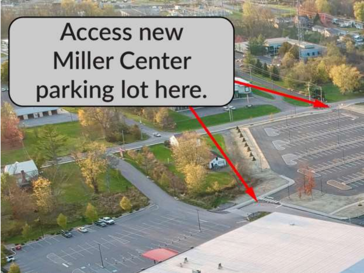
Larger view of new parking lot access.
